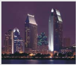
Building Outside Lighting
