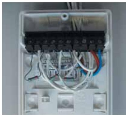
Typical simple E-Line wiring
